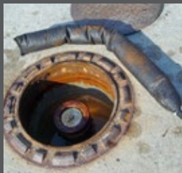
Remove saturated sock & replace if necessary
