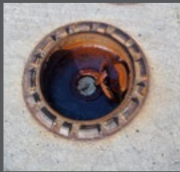
Water overflow causes cap release & leakage into tank
